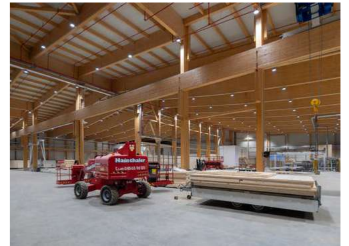
Penzkofer Bau, Germany, Photo: Molto Luce
